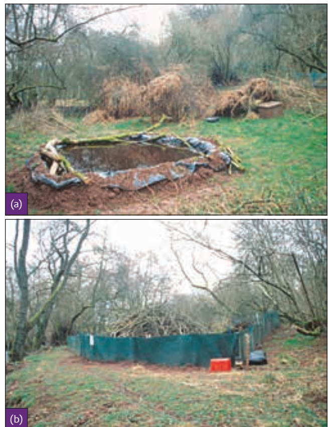
9.6 Soft-release enclosure for otters. (a) Construction of the pool and artificial holt. (b) The fence used for the enclosure. The fence comprises an electric mesh fence (such as that used for chickens) with a plastic windbreak on the outside, so that the otter cannot see outside the pen.
